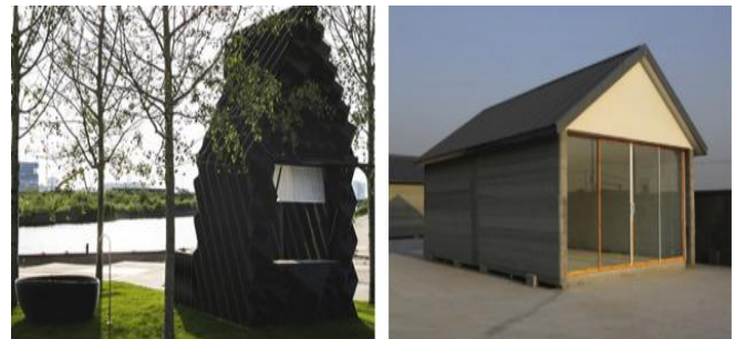
Fig. 4: (a) First 3D printed house (taken from Dus Architects [50]) (b) 3D printed house (taken from P. Wu et al [3])
