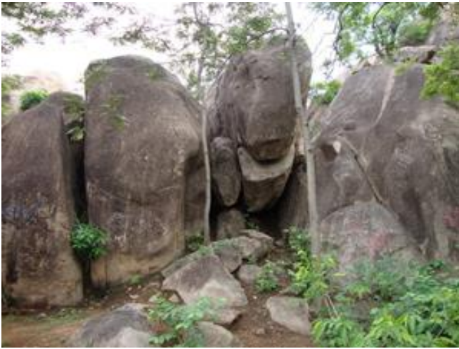
Fig. 14: Cracks developed within the rocks and they are widening day by day due to weathering, both physical, chemical and biological weathering.
